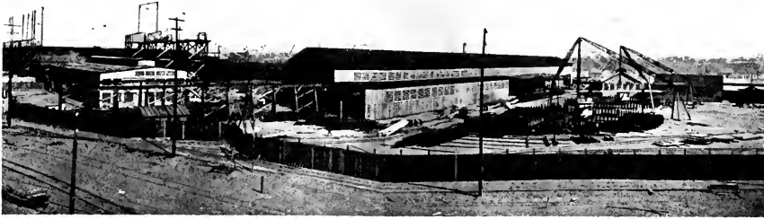
The stiff leg-derrick cranes covering the plate and shape storage space at the Duthie plant.
